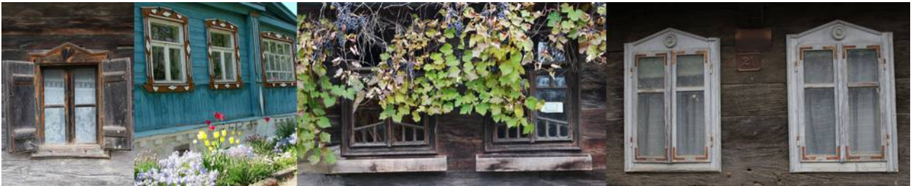
A selection of windows from local traditional wooden houses
