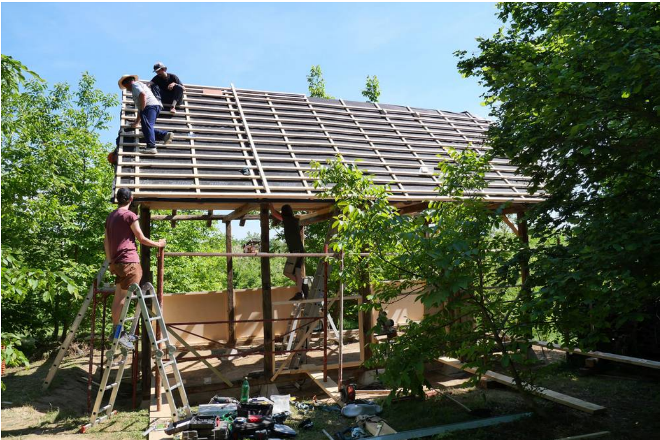
Building the 1st house in the food forest!
