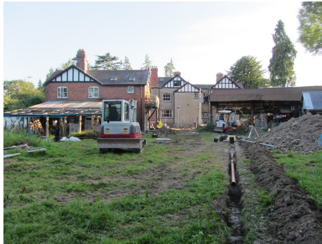
The sewage outflow pipe goes into the ground.
