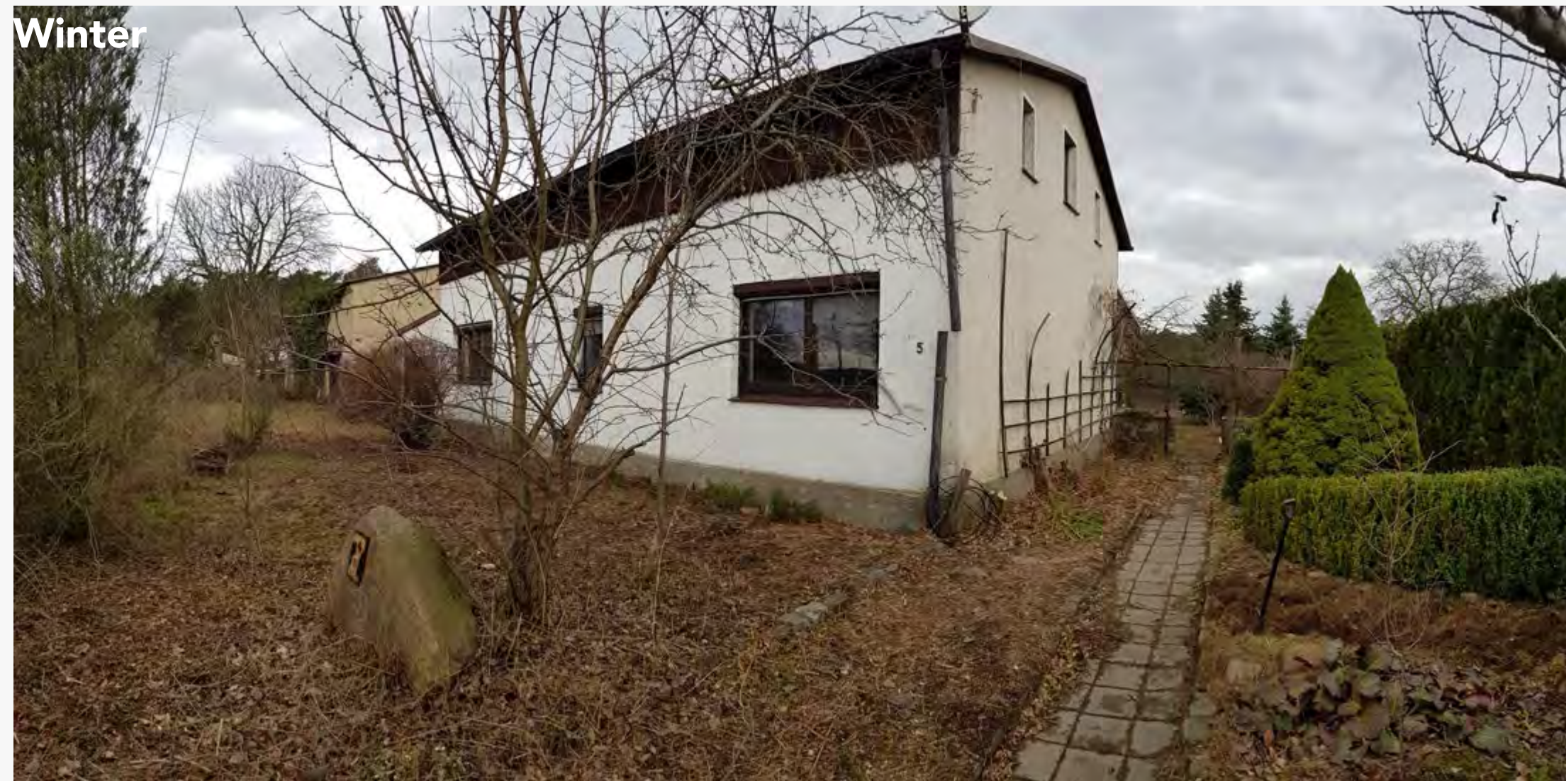
Standing in the frontyard at south-east border, looking northwest at Ankes' house in winter
