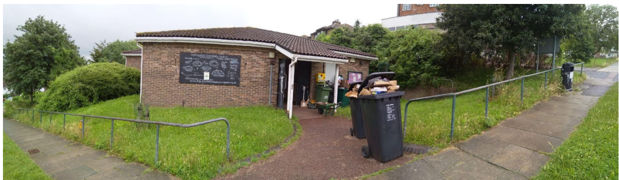
Panoramic view of the front garden. This shows the problem with recycling and waste bins at the entrance.
